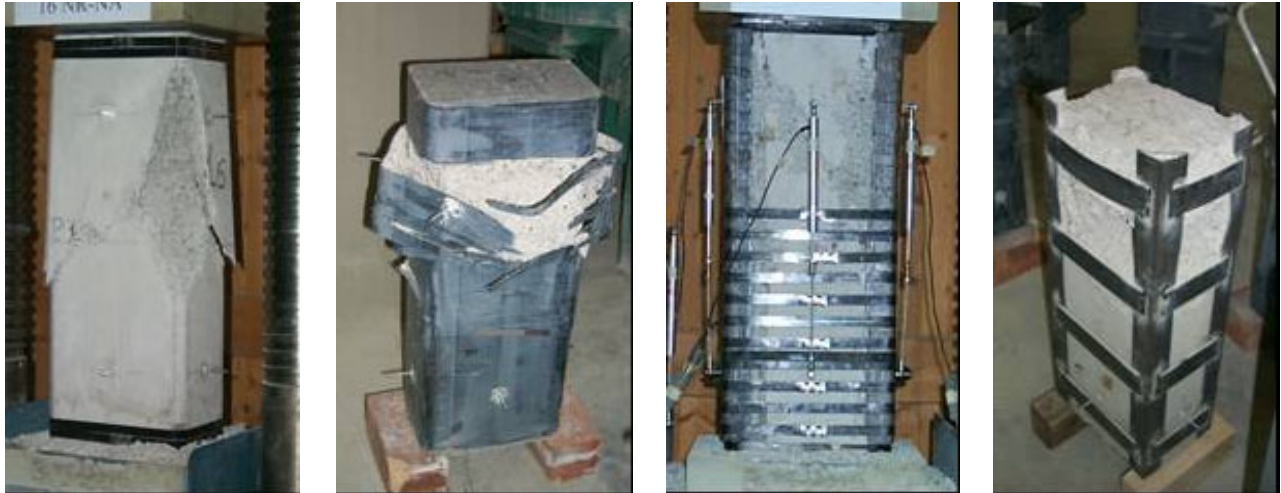
Fig. 7: Typical failures observed in the unreinforced columns
